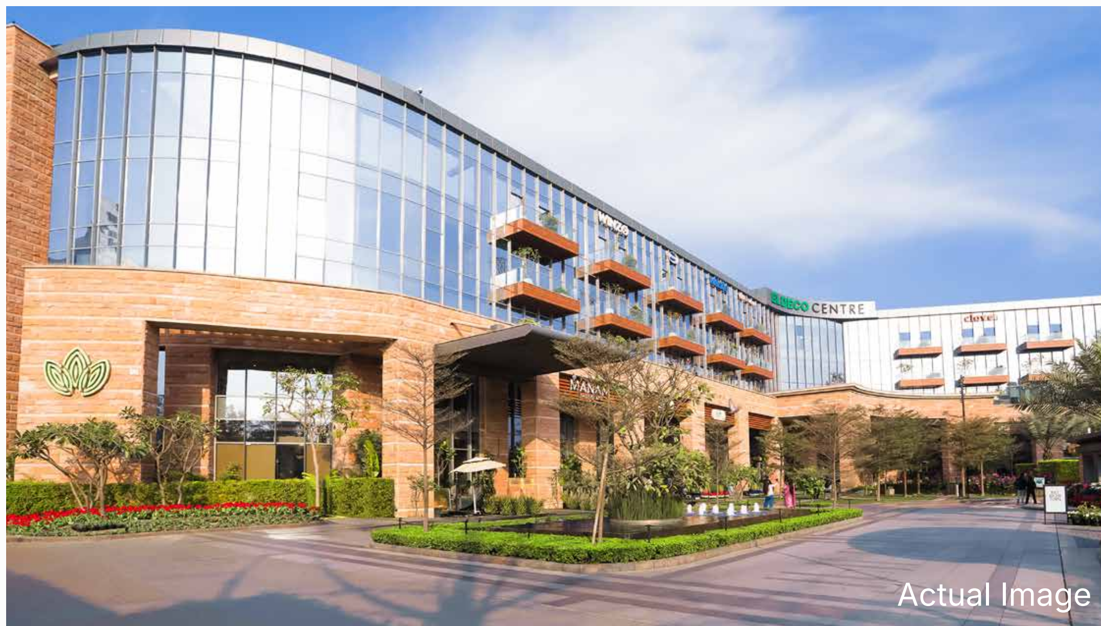
Eldeco Centre, Malviya Nagar
